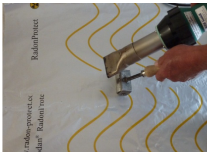
RadonProtect Foil, welding by hot air gun
